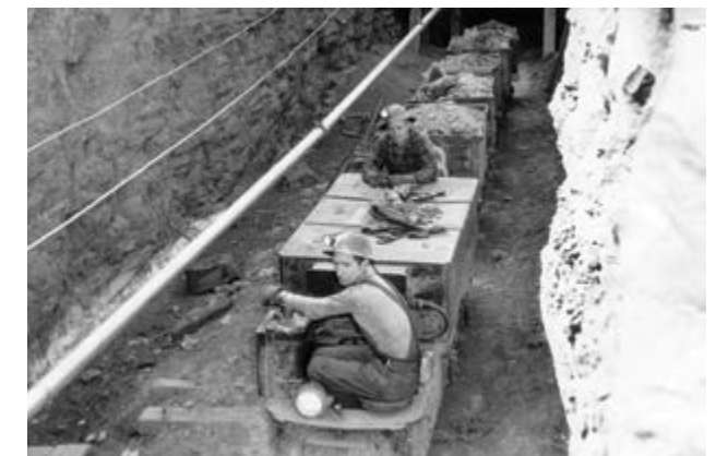
Ore cars bring uranium out of the Radium King Mine on the Colorado Plateau.
