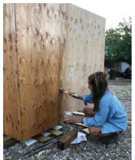
Jessie Page coating the exterior of the dehydrator with linseed oil to help protect it from the elements
